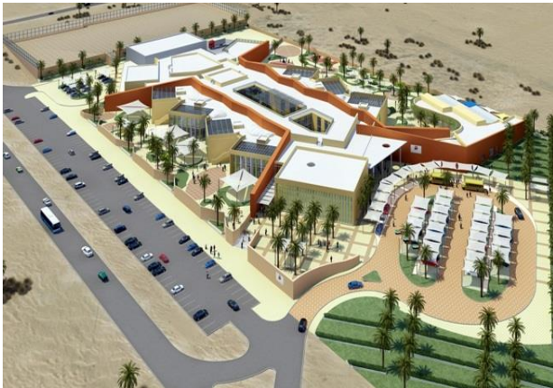
CLIENT: Musanada CONSULTANT: KEO International Consultants CONTRACTOR: Al Fara'a General Contracting Co. L.L.C
