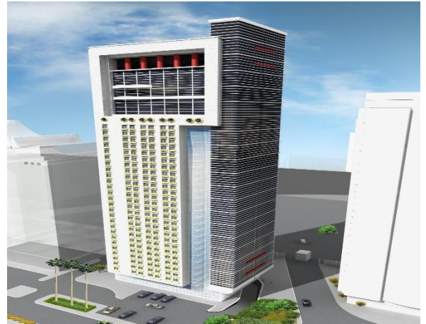
CLIENT: International Capital Trading CONSULTANT: Bainona Consulting Engineering CONTRACTOR: Seidco General Contracting
