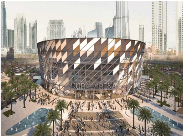
CLIENT: Meraas Holding CONSULTANT: Dar Al Handasah CONTRACTOR: Al Shafar General Contracting
