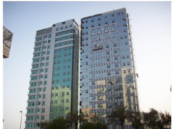
CONSULTANT: Heberger Engineering Consulting Engineers CONTRACTOR: Bin Hermal General Contracting L.L.C
